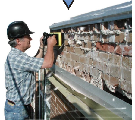
GPR in use on masonry wall
