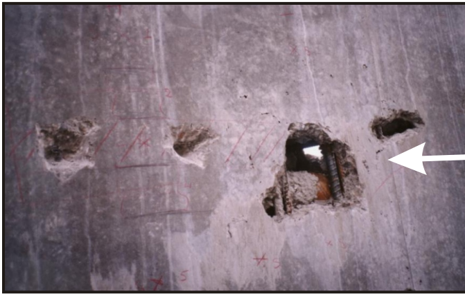
Extent of honeycombing evaluated around duct of precast bridge beam
