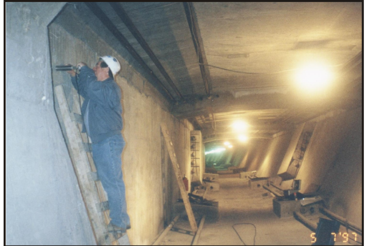
Testing post-tension ducts for partial filling
