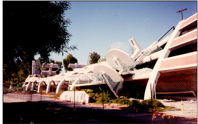
UCLA parking garage after 1994 California earthquake
