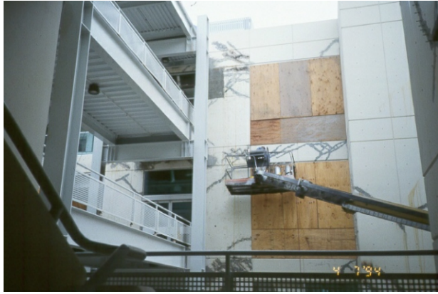
Measuring crack depths
