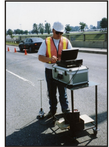
Testing a bridge deck for delamination
