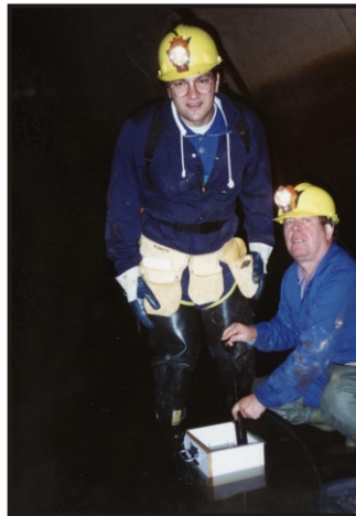
Testing aqueduct concrete below water level
