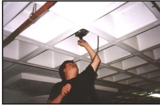
Testing parking garage soffit for bond to topping
