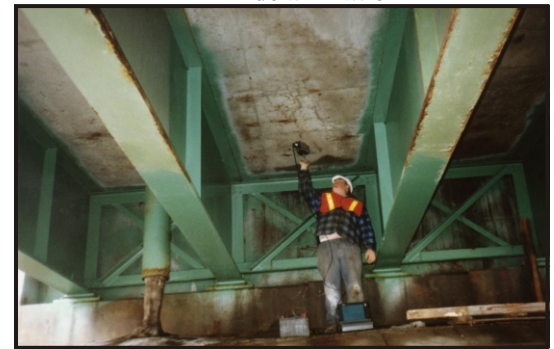
Testing bridge soffit for defects
