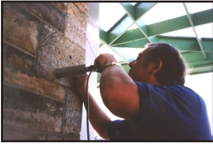
Testing masonry for bond to concrete
