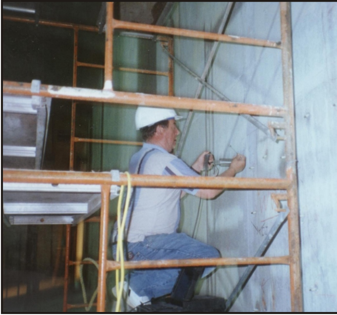
Testing joints with impact-echo equipment
