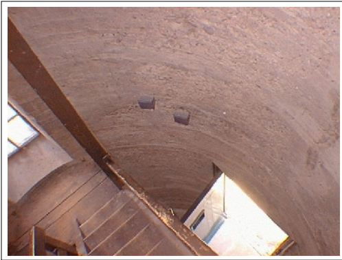
Views of the inside concrete shell of the monument
